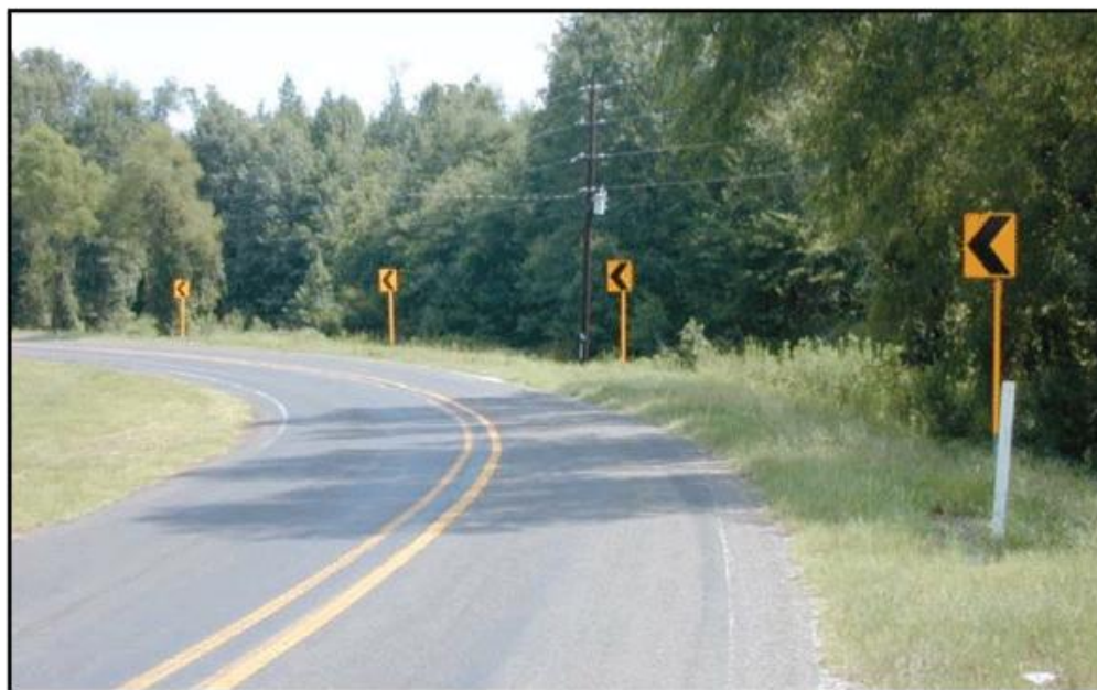
Figure 46: Enhanced Delineation Chevron Signage
