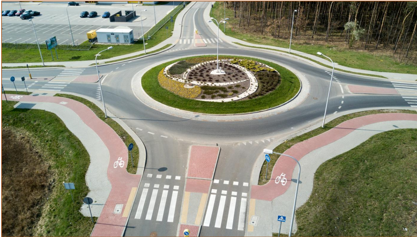
Figure 44: Roundabout with Multimodal Facilities
